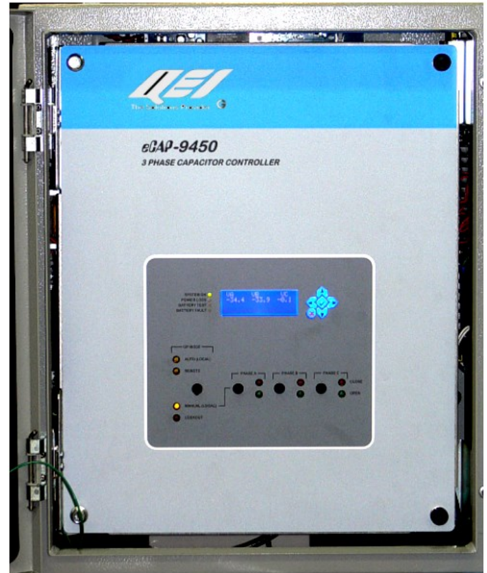
Front Panel LED Readout Permits Quick Review of Controller Operation Without the Need for a Laptop
